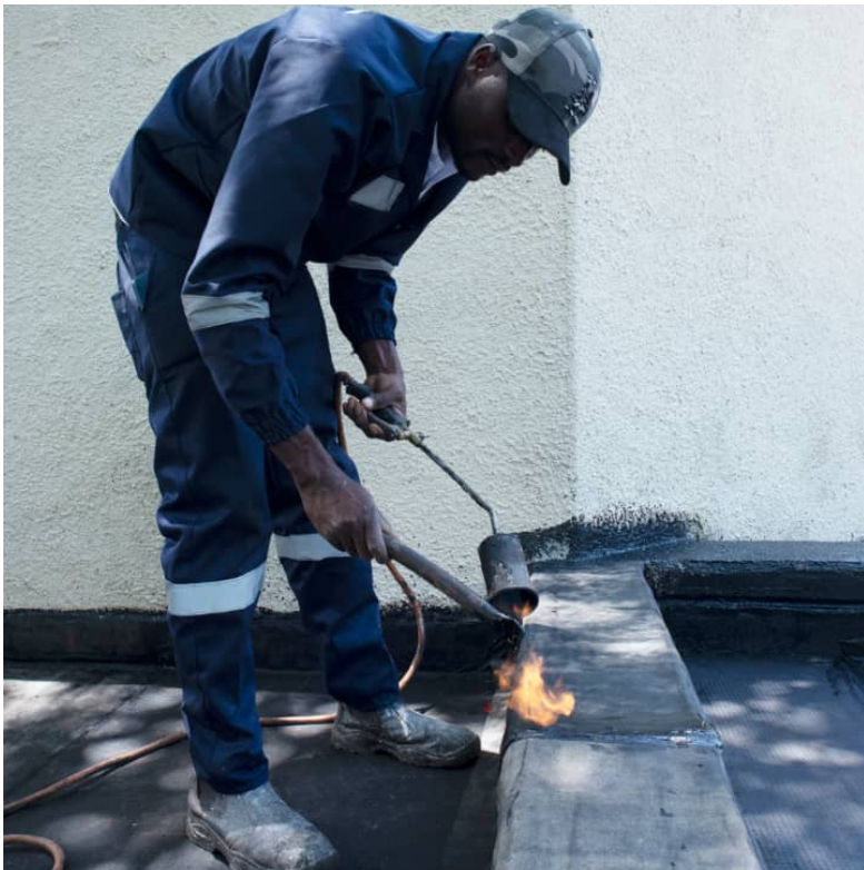
Switzerland Embassy Concrete Deck torch-on waterproofing, Belgravia, Harare
