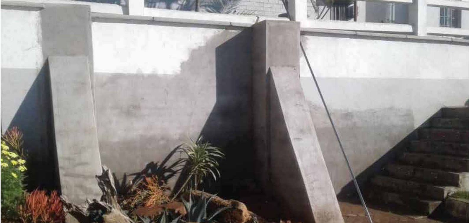
Trek Service Station Buttress Walls, Charter Road, Harare
