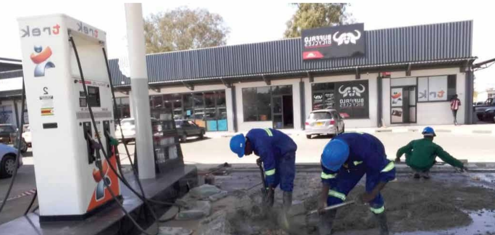
Trek Service Station cut off drain, Msasa, Harare
