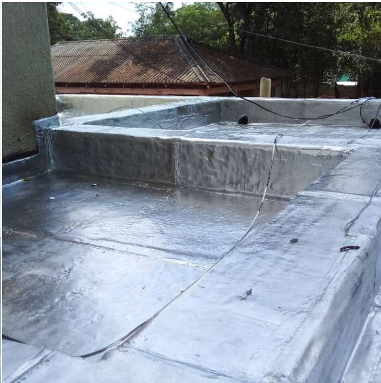
Switzerland Embassy Concrete Deck torch-on waterproofing, Belgravia, Harare
